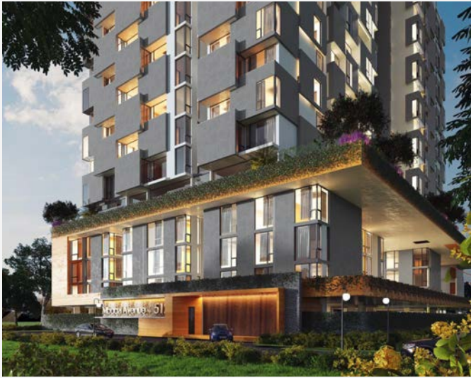
Mbaazi View Apartments
